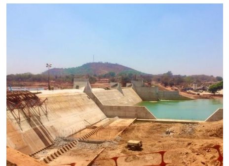
The new dam
