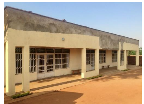
Our new building getting a lick of paint
