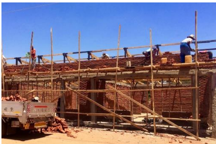
Our new home under construction
