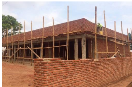
Progress in late November
