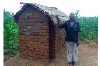
New Pit Latrines
